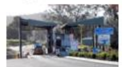
Weighbridge at entrance to WMC
